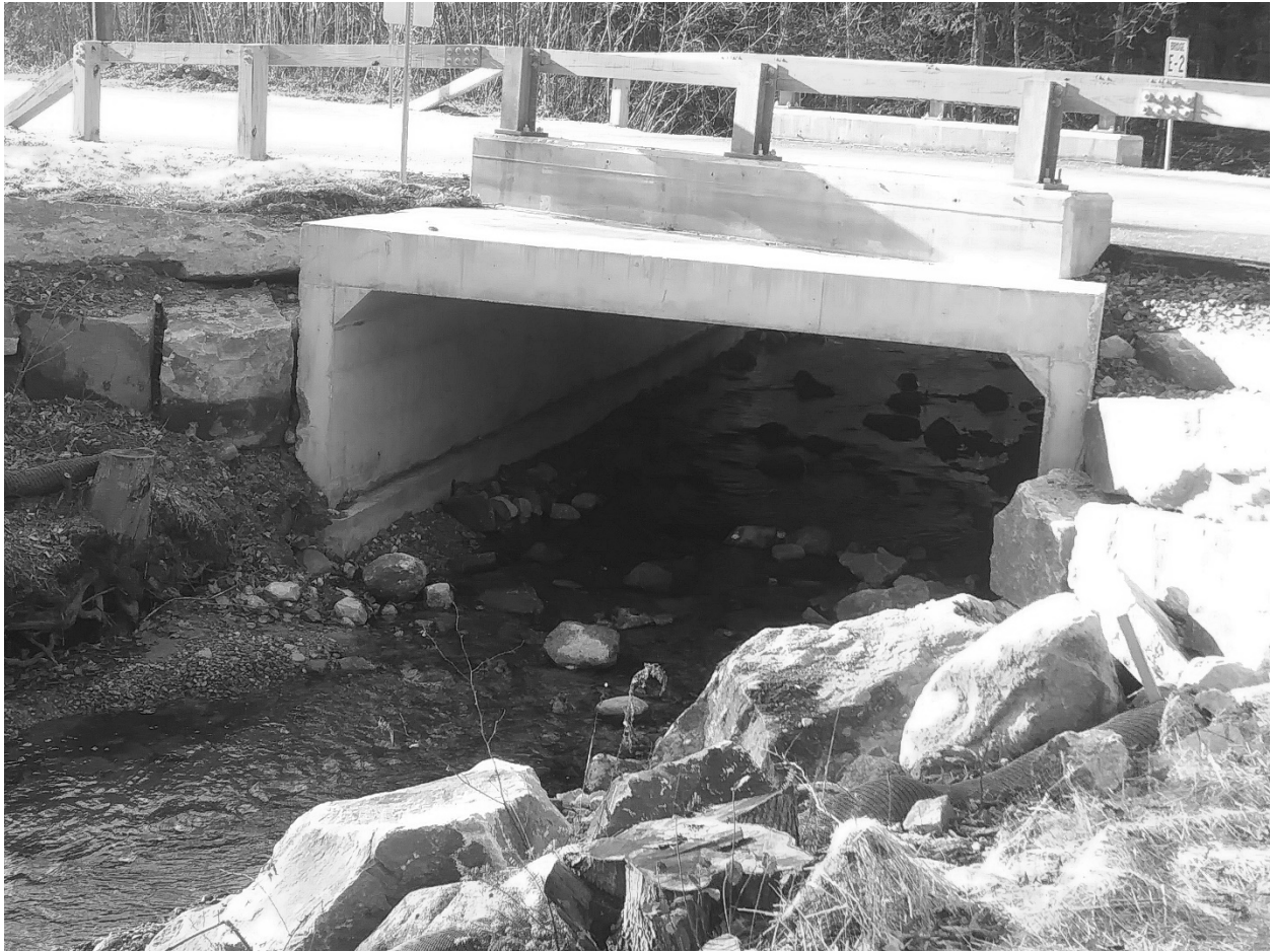
Durand Road West Bridge
